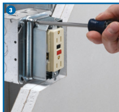
Re-tighten... Adjustment screws.
