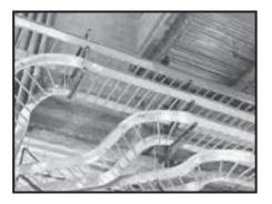
As a lighting support system, metal framing helps assure proper alignment over long spans. As a raceway system, channel offers an opportunity to reduce construction costs through more efficient use of installation labor. The exceptional versatility of channel gives contractors more flexibility in solving miscellaneous problems which may arise at the job site.
